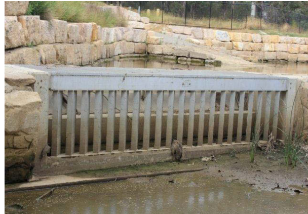
Photo 4: Offline tilting weir with pollution deflector
