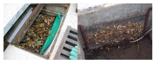
Figure 6. Leaf Accumulation in Pre-Filtering Devices (Left: Asquith; Right: Kiama)
