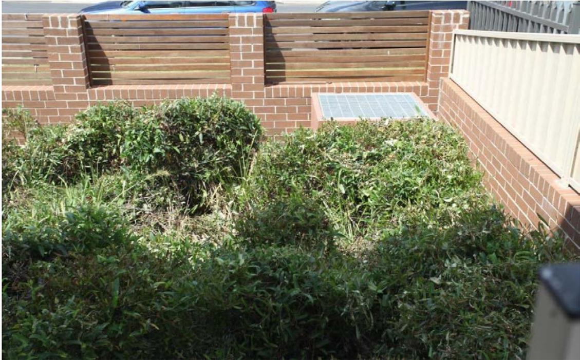
Plate 2 showing a vegetated stormwater system which is not maintained and which sterilises the limited open space on this development. Image courtesy Steve Araj.
