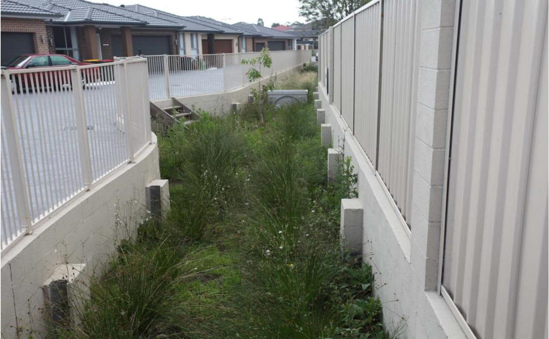
Plate 1 showing how bioretention and OSD are frequently shoe horned into developments and how safety fences isolate them rather than facilitating integration into the development. Image courtesy Steve Araj.
