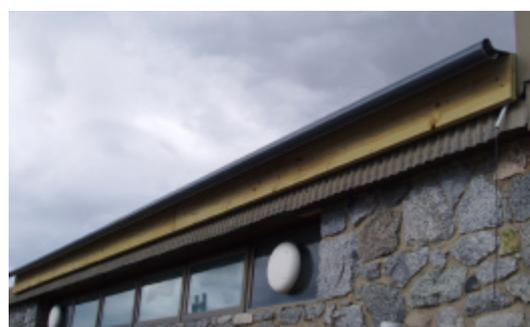
**Figure 3.** Priority Alpine roof gutter fitted to existing roof
