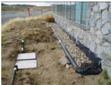
**Figure 5.** Ground collection component of trial showing dual collection sump on LHS
