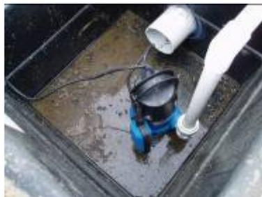
**Figure 6.** View inside one of the collection sumps showing pumping arrangement
