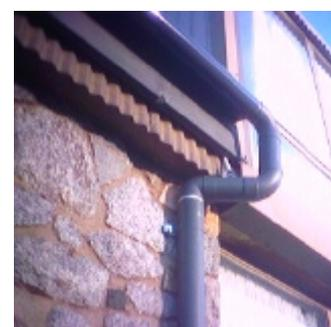
**Figure 4.** Downpipe conveying flow into collection sump
