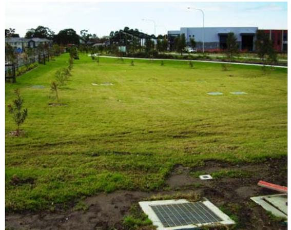
Plate 3 – Basin C with 800 kL stormwater storage beneath
